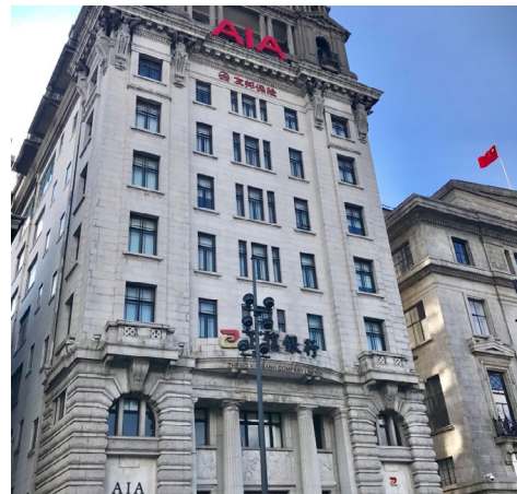
The AIA building on Zhongshan Road, Shanghai
